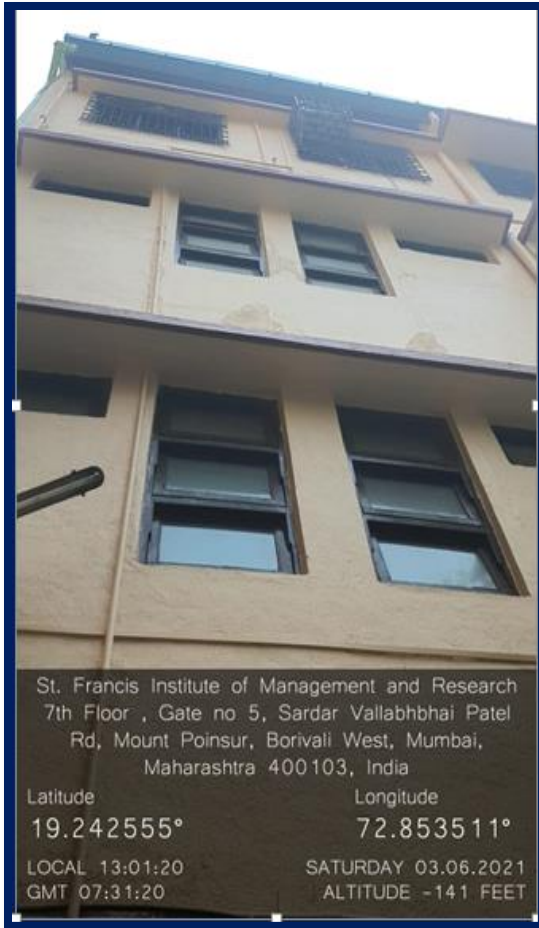
Water gets stored at the rooftop
