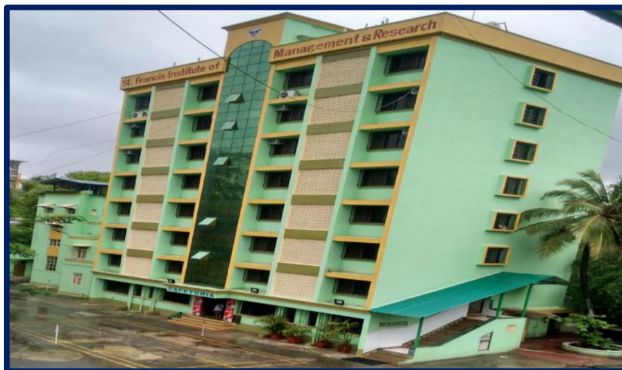
SFIMAR Hostel Building
